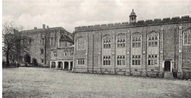
Upper Yard and Old Assembly Hall
